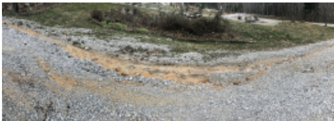
Ruts forming along the driveway between our neighbor's and our property.
