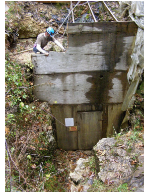
Top and Above: Dismanteling the duct and the wooden façade.
